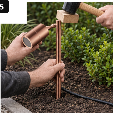
INSERT STAKE / KEEP PLUMB / SET AIM
