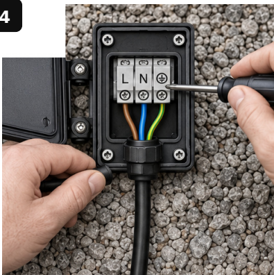
CONNECT IN ACCESSIBLE IP-RATED JUNCTION
