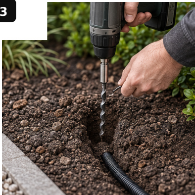
PREPARE NARROW PILOT / ROUTE CONDUIT
