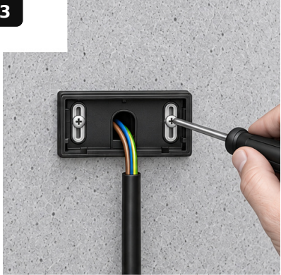
DRILL / ANCHOR / FIX SMALL PLATE TO WALL
