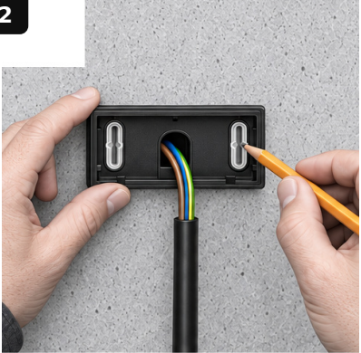
LEVEL SMALL FIXING PLATE / MARK ANCHORS
