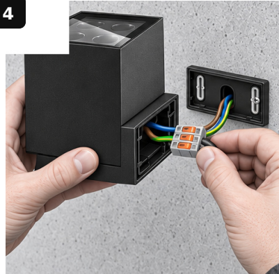
CONNECT L-N-PE / SEAL CABLE ENTRY
